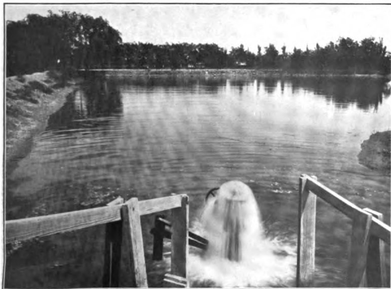
B. ARTESIAN WELL AND RESERVOIR EAST OF SOUTH SPRING, NEW MEXICO.
